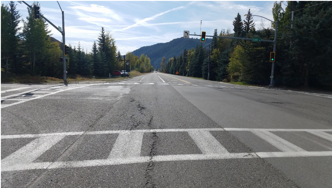
Photo 3: Looking south east on SH-75, from Saddle Rd. Photo taken on 7/8/2019.
