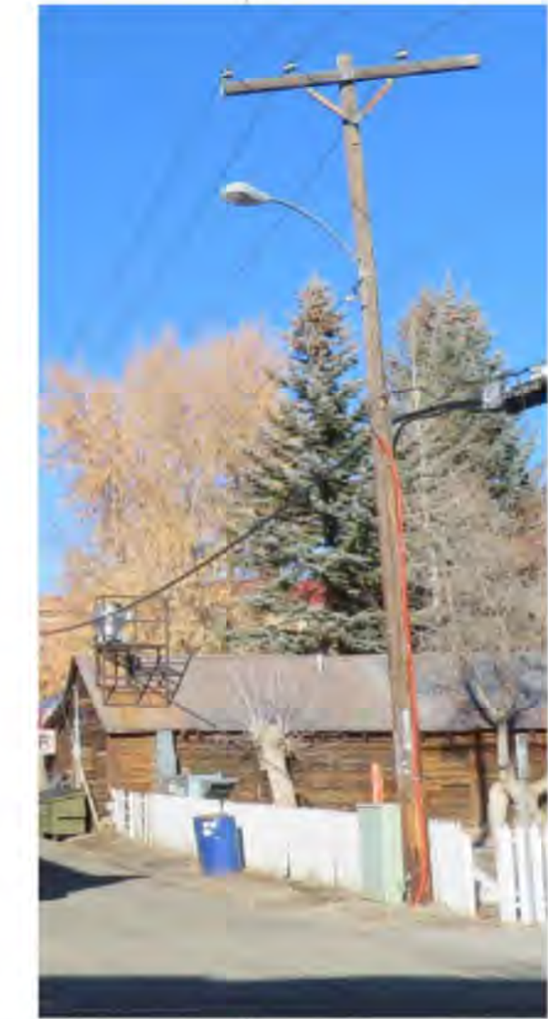
Approximate location of power pole-mounted light Fixture height: ±23'-0"
