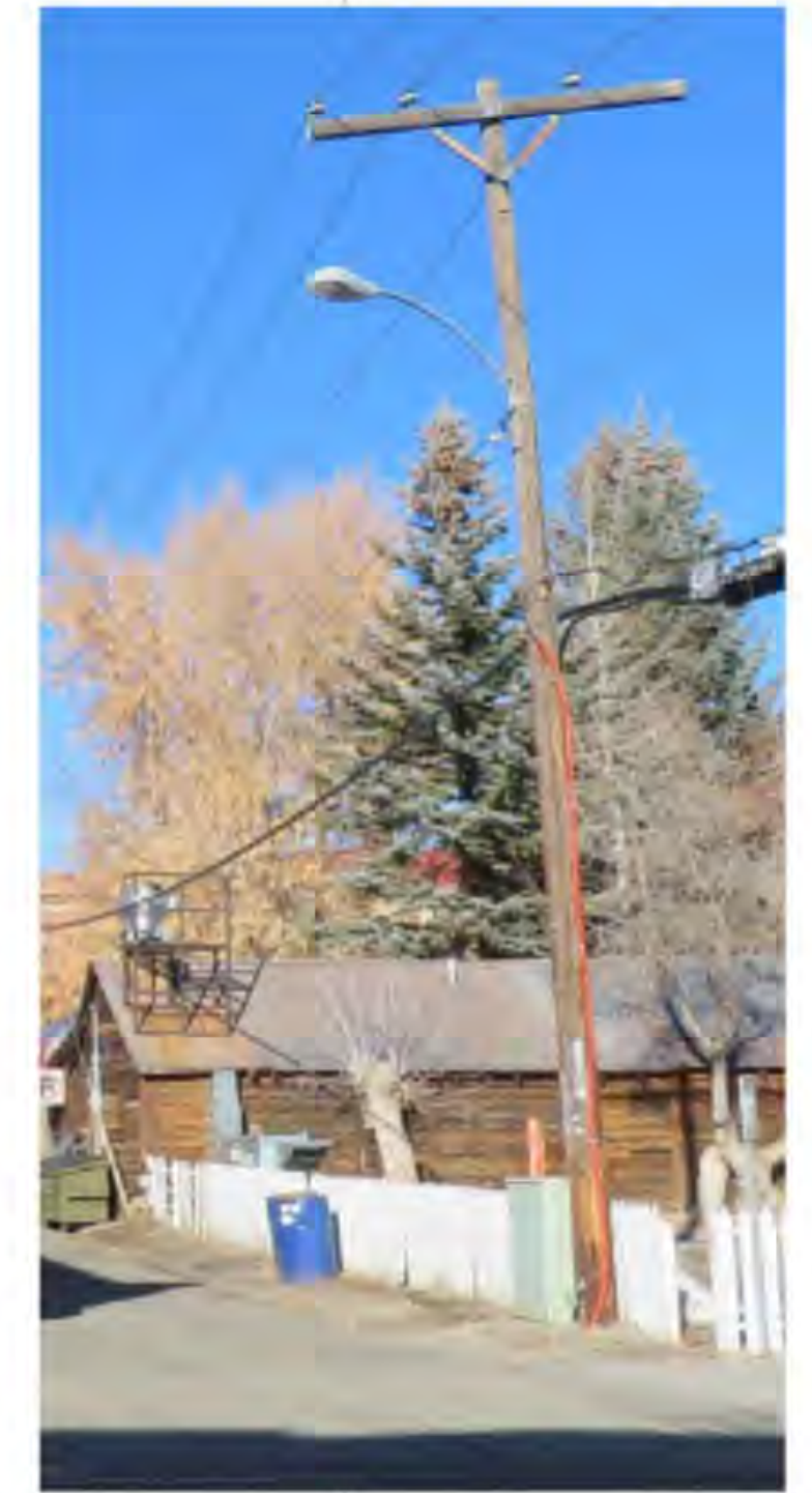
Approximate location of power pole-mounted light Fixture height: ±23'-6"
