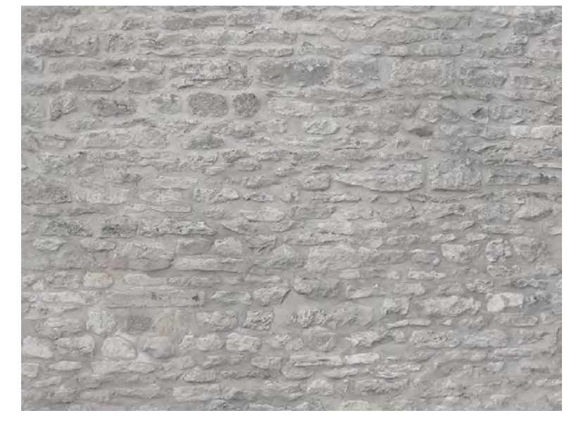
PARGED FIELD STONE: WALLS
