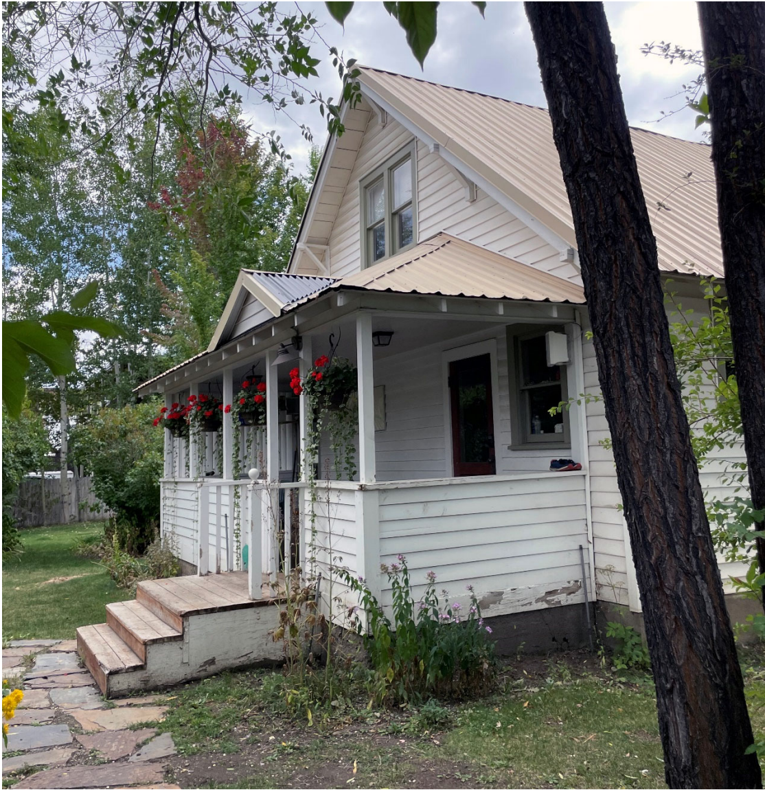
Photo C: Back Porch, Northeast side
