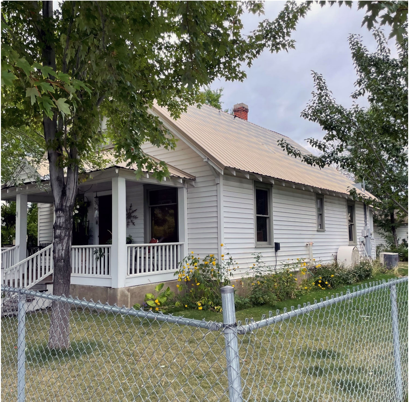
Photo B: South side of building
