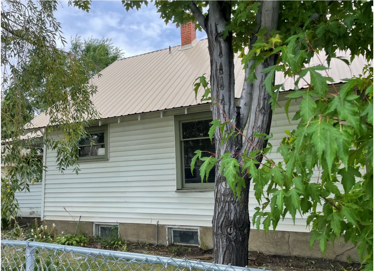
Photo D: North Façade
