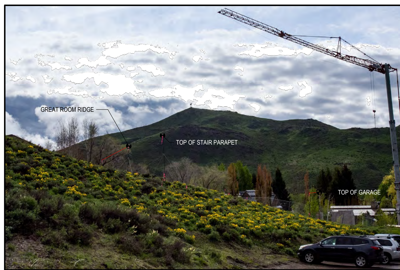
EXHIBIT A: FROM NEIGHBORING DRIVEWAY
