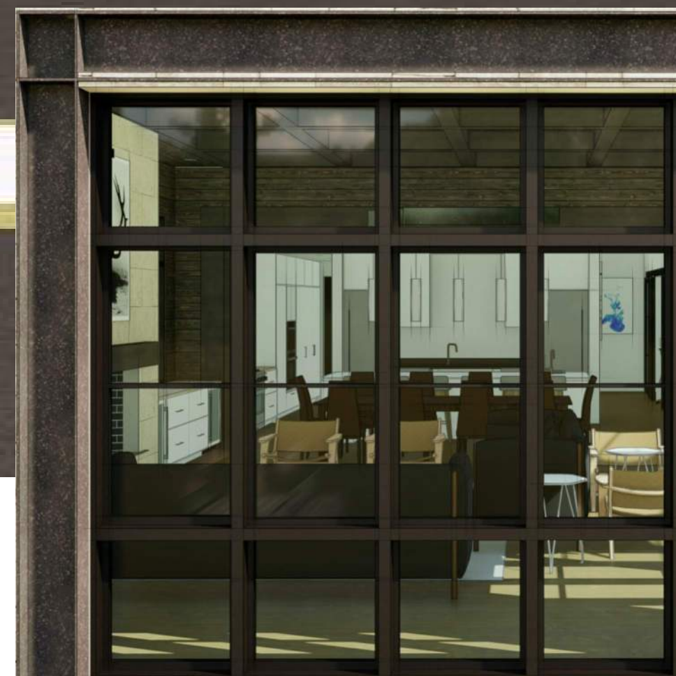
WINDOWS: ALUMINUM CLAD WOOD WINDOWS COLOR: DARK BRONZE
