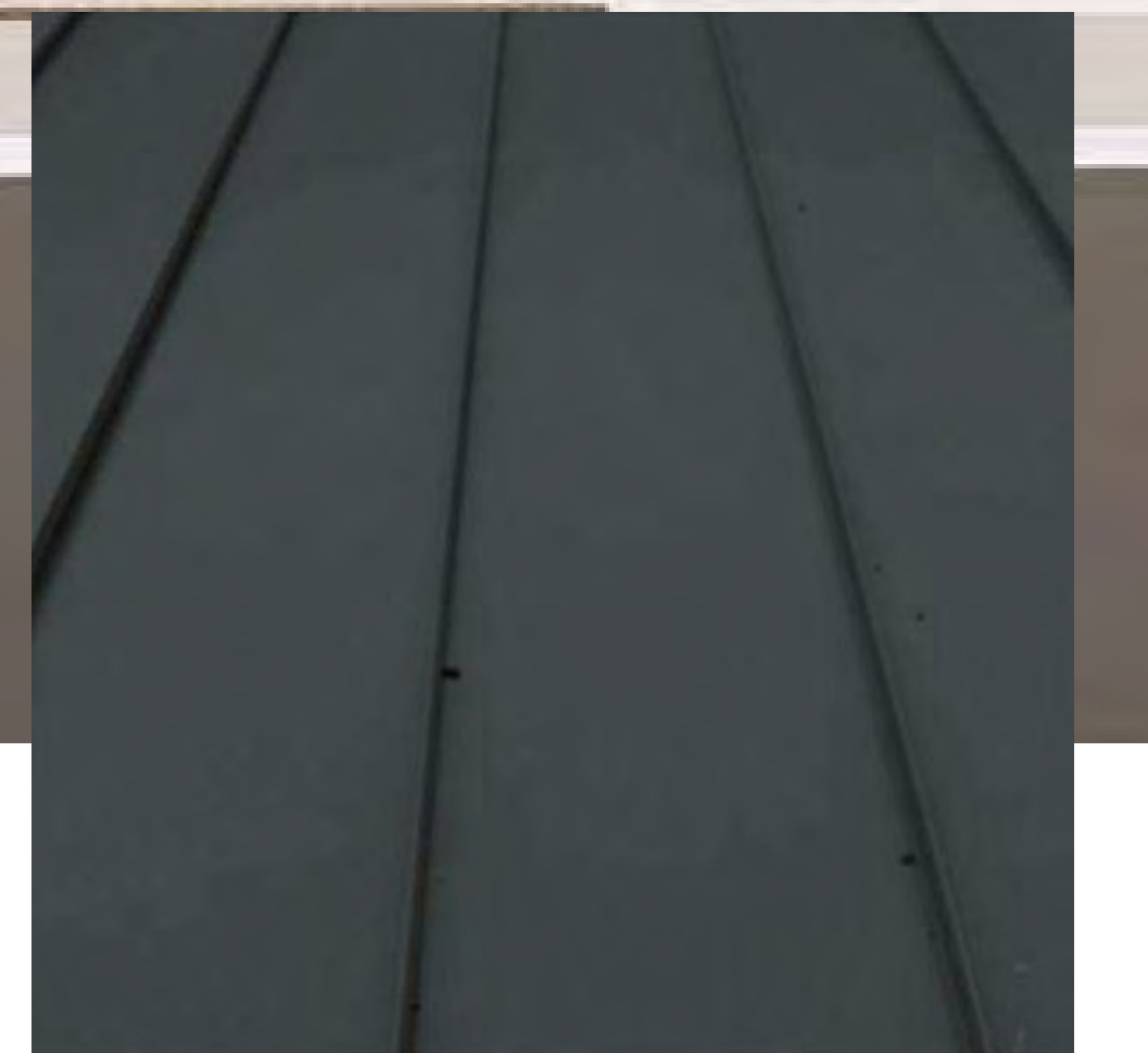
METAL ROOFING ON ELEVATOR:
