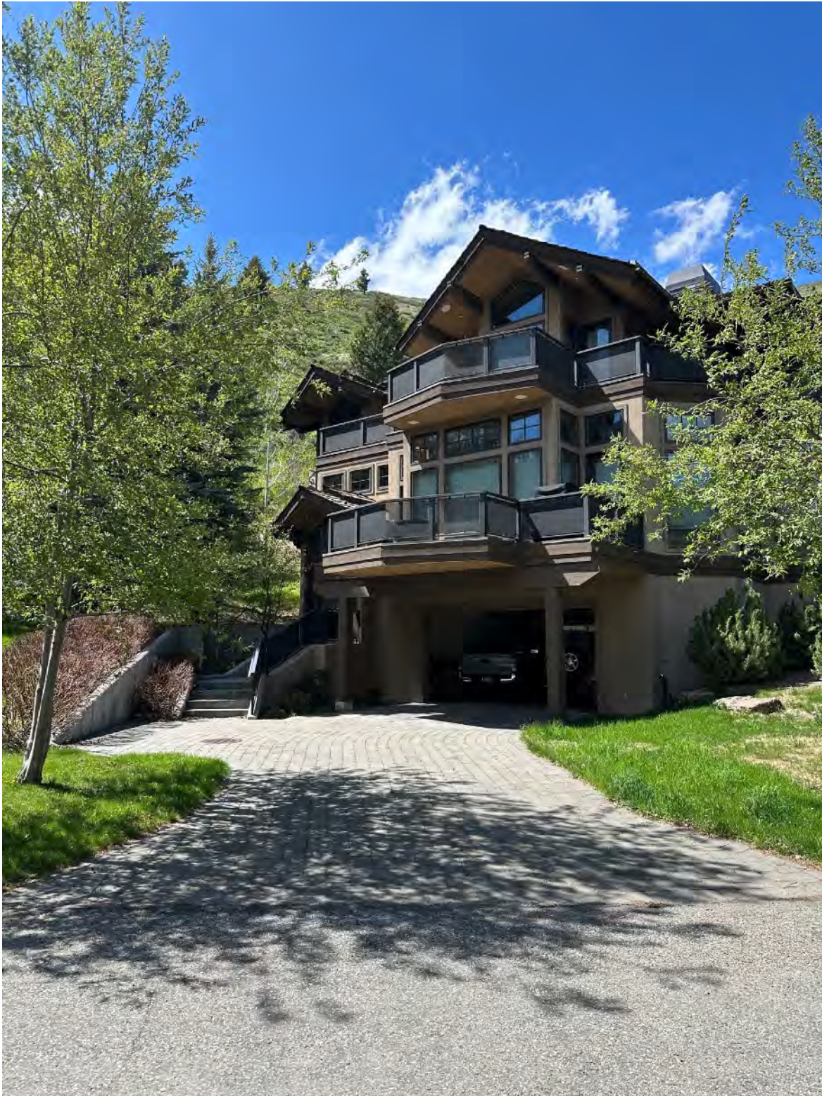
394 Sage Rd. Architect-designed home. Architectural features / interest, upper floors stepped back, no flat facade. Unit 400 would start approximately in-line with catch basin on left side of driveway.
