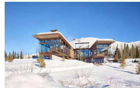
Bigwood Residence East & Sun Valley Rd
