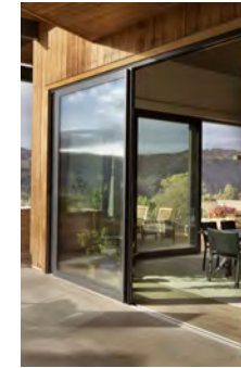
9 MULTI-PANEL SLIDING GLASS DOORS (OPERABLE WALL)
