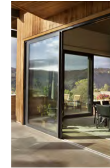
9 MULTI-PANEL SLIDING GLASS DOORS (OPERABLE WALL)
