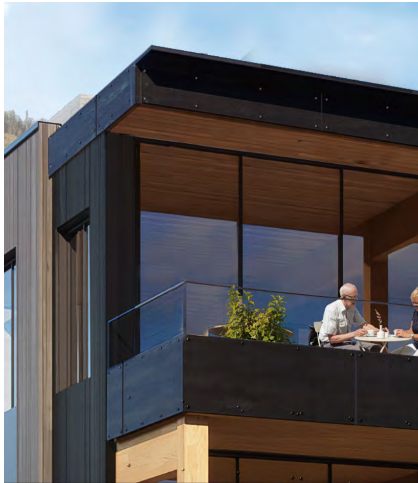
OPEN JOINT PAINTED STEEL PLATE CLADDING WITH EXPOSED FASTENERS
