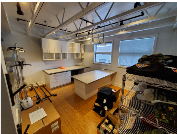
Upper Level Office
