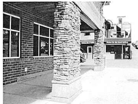
Unequal sides of columns are discouraged
