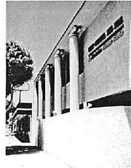
Blank walls and facades that do not clearly delineate each floor of the building are prohibited:
