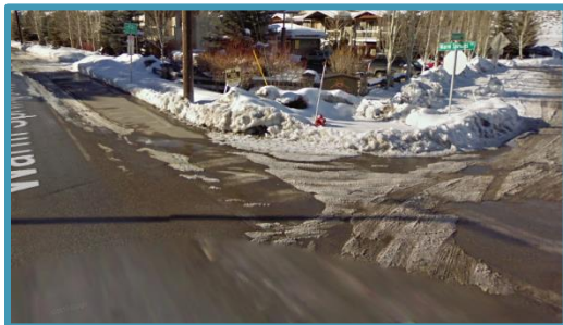
Cycle track adjacent to Warm Springs Road and intersection crossing
