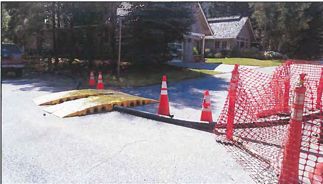
CROSSING OF TEMPORARY LINE IN ASPEN DRIVE
