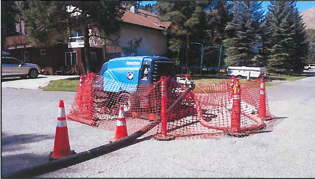
TEMPORARY PUMP SETUP IN ASPEN DRIVE
