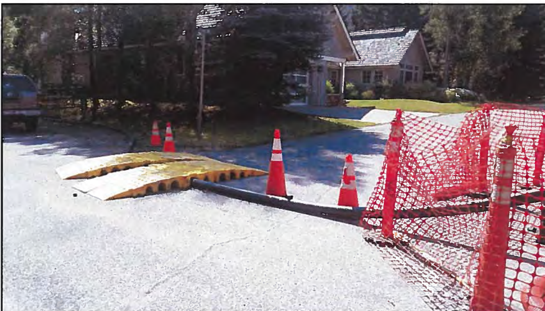
CROSSING OF TEMPORARY LINE IN ASPEN DRIVE
