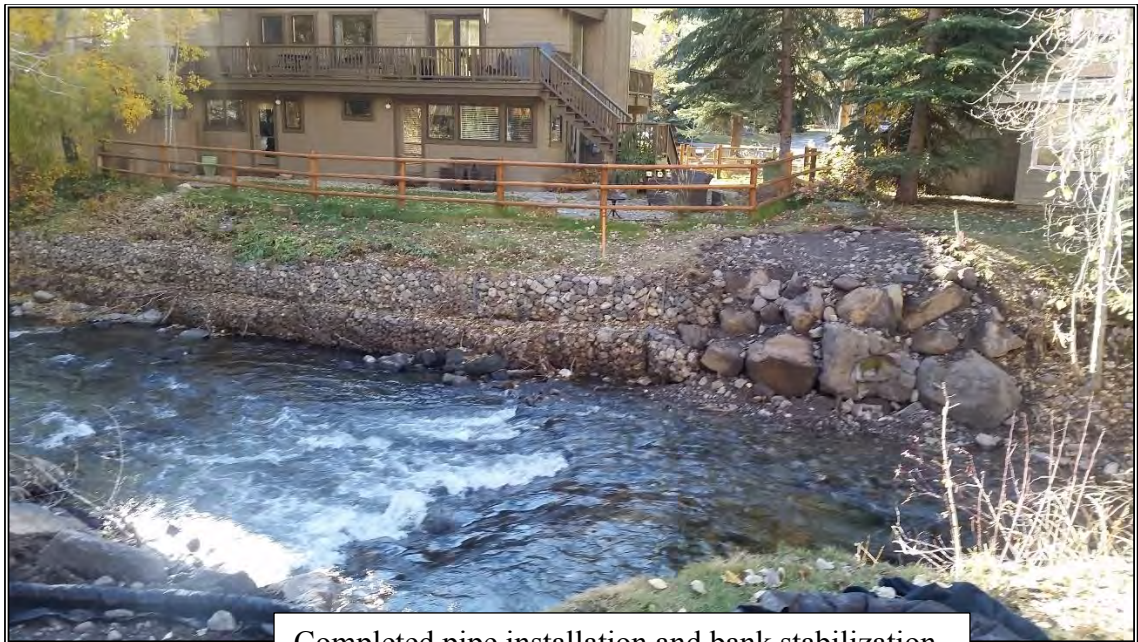
Completed pipe installation and bank stabilization
