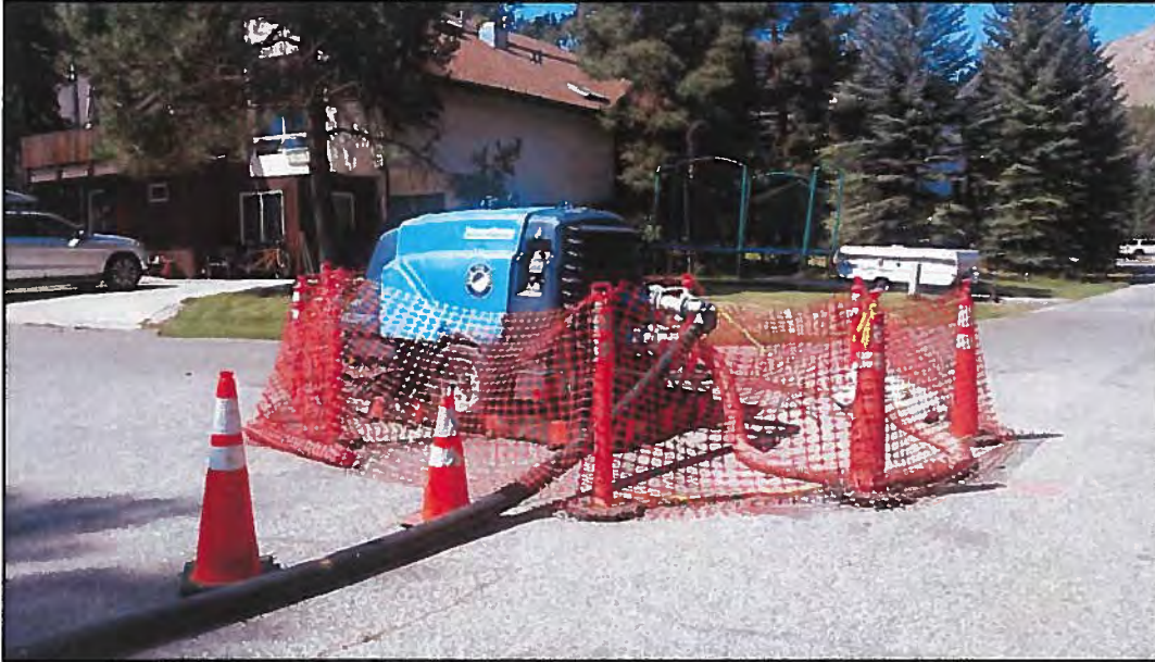
TEMPORARY PUMP SETUP IN ASPEN DRIVE
